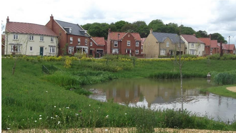
SUDS drainage pond at Grey Towers Village, Middlesbrough
